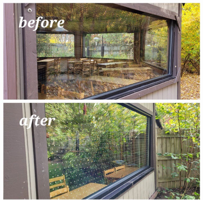
Bird observatory windows before and after the installation of Feather Friendly bird collision deterrent markers on the windows.
